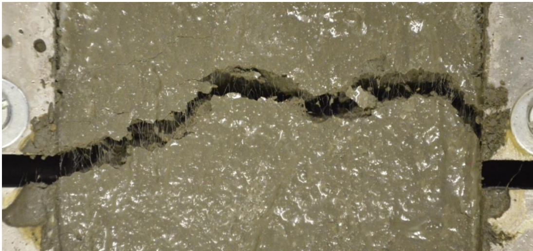
Direct tensile test on fresh concrete clearly showing the fibres bridging the crack even after extensive crack opening.
